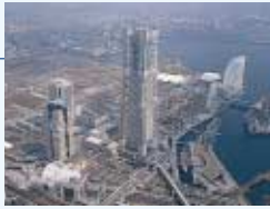
The construction of facilities was progressing steadily (1994).
